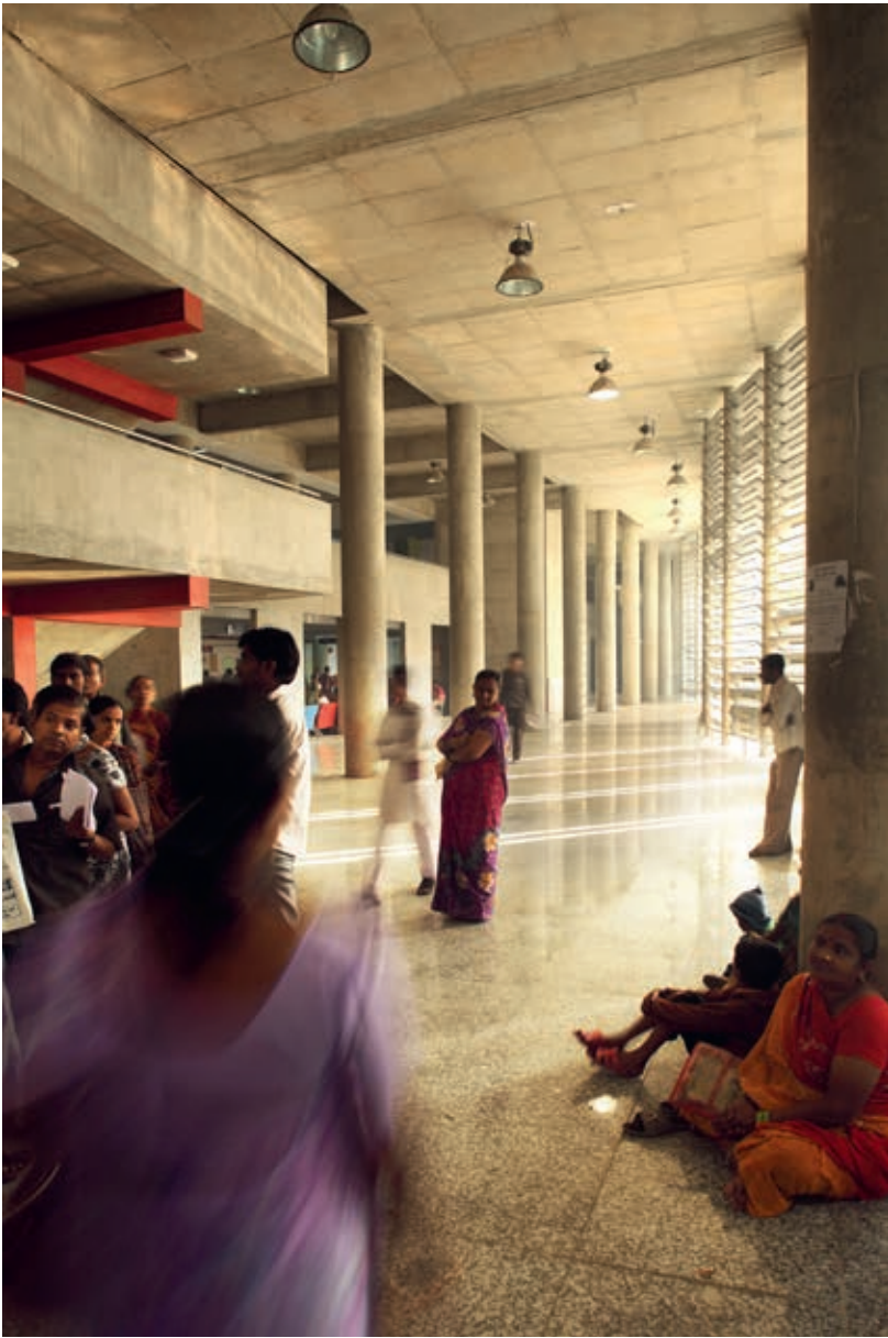
Opposite, and above left and right: Negating the need for air-conditioning, the louvers create a draft and comfortable ambient temperature in the Outpatient Department. Earmarked funds were instead utilized in the development of an 80,730-square-foot (7,500-square-meter) garden that is also open to public.
